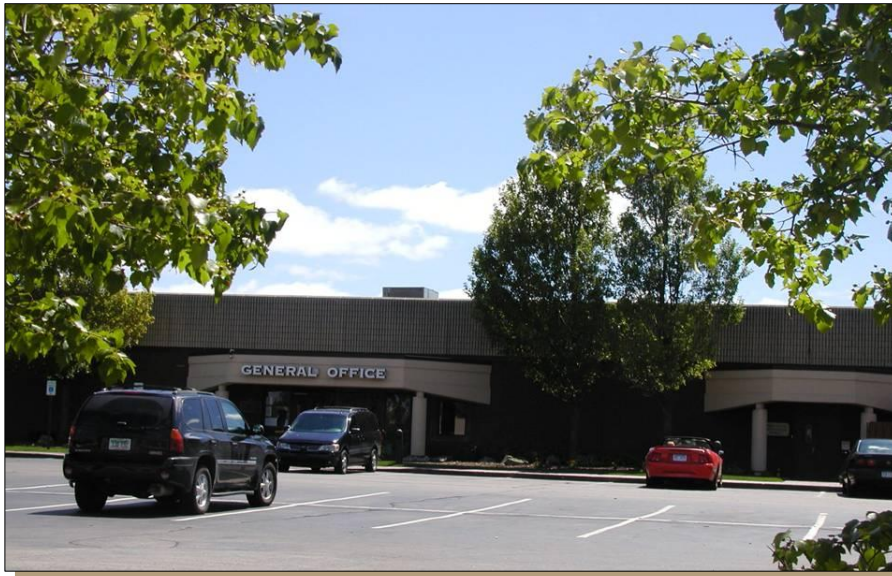
The north wall (building entrance) today.
